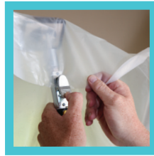
clip plastic onto quick clip
